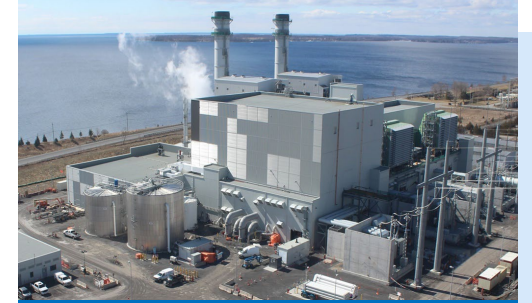
4. Napanee Generating Station 2020-2060 Capacity 900 MW
