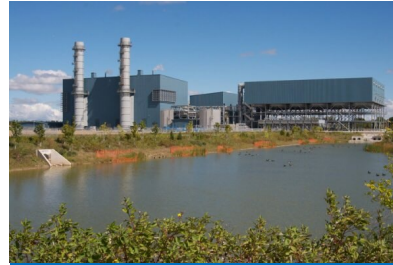
2. Halton Hills Generating Station 2010-2050 Capacity 683 MW
