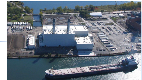
3. Portlands Energy Centre 2009-2049 Capacity 562 MW
