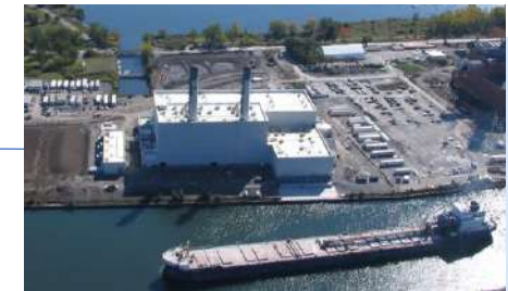
3. Portlands Energy Centre Capacity 562 MW
