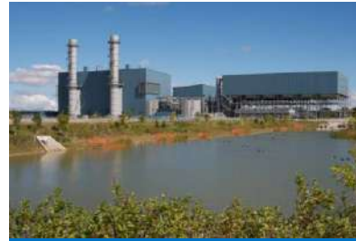
2. Halton Hills Generating Station Capacity 683 MW
