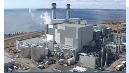
4. Napanee Generating Station Capacity 900 MW
