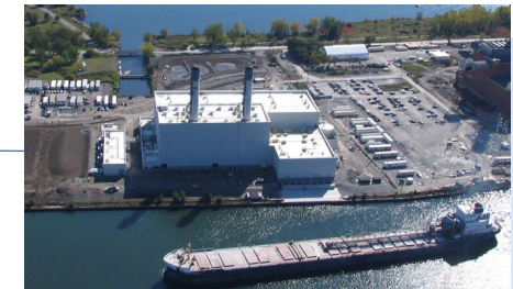
3. Portlands Energy Centre Capacity 550 MW
