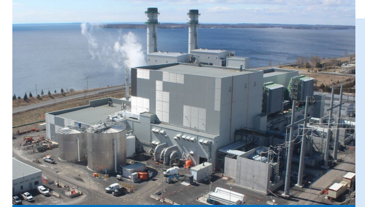
4. Napanee Generating Station Capacity 900 MW
