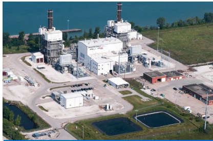
1. Brighton Beach Generating Station Capacity 570 MW
