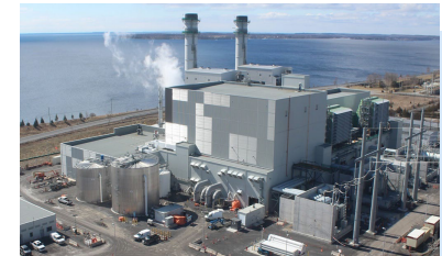
4. Napanee Generating Station 2020-2060 Capacity 900 MW
