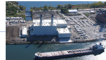
3. Portlands Energy Centre 2009-2049 Capacity 562 MW
