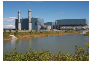
2. Halton Hills Generating Station 2010-2050 Capacity 683 MW
