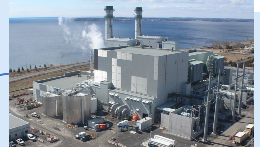
4. Napanee Generating Station Capacity 900 MW
