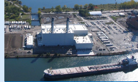
3. Portlands Energy Centre Capacity 550 MW
