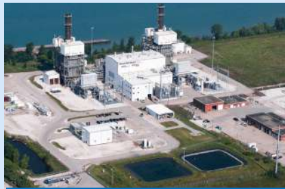
1. Brighton Beach Generating Station Capacity 570 MW
