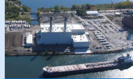
3. Portlands Energy Centre Capacity 550 MW
