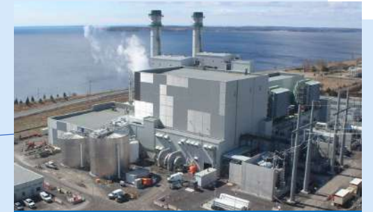
4. Napanee Generating Station Capacity 900 MW
