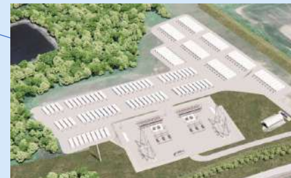
5. Napanee BESS Phase 1 Capacity 250 MW
