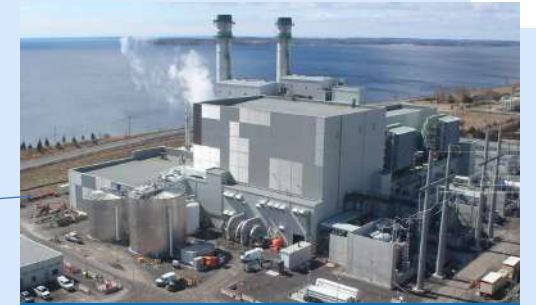
4. Napanee Generating Station Capacity 900 MW
