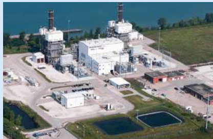
1. Brighton Beach Generating Station Capacity 570 MW
