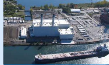
3. Portlands Energy Centre Capacity 550 MW
