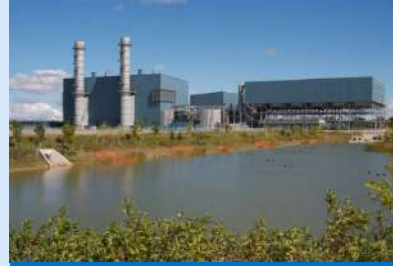
2. Halton Hills Generating Station Capacity 683 MW
