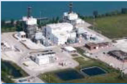
1. Brighton Beach Generating Station Capacity 570 MW
