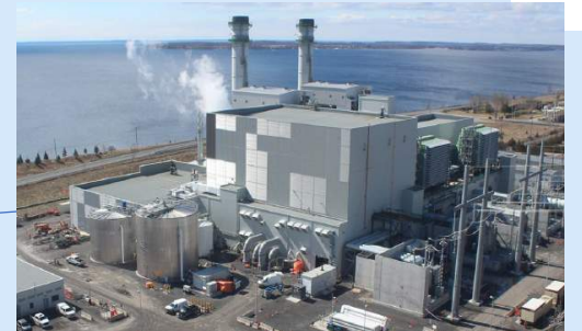
4. Napanee Generating Station Capacity 900 MW
