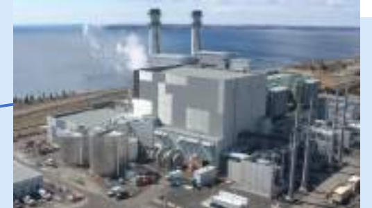
4. Napanee Generating Station Capacity 900 MW
