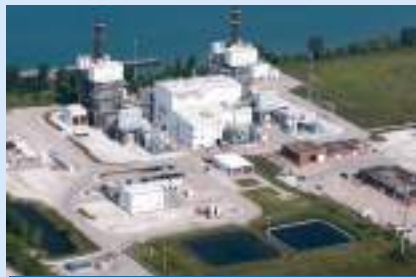
1. Brighton Beach Generating Station Capacity 570 MW
