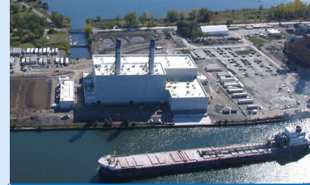
3. Portlands Energy Centre Capacity 550 MW
