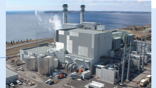
4. Napanee Generating Station Capacity 900 MW
