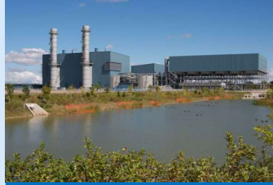
2. Halton Hills Generating Station Capacity 683 MW
