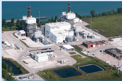
1. Brighton Beach Generating Station (570 MW)
