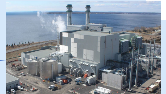
4. Napanee Generating Station (900 MW)
