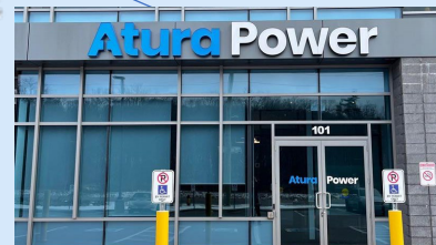
6. Oakville Head Office
