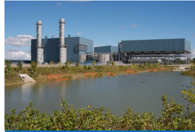
2. Halton Hills Generating Station Capacity 683 MW
