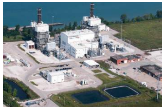
1. Brighton Beach Generating Station Capacity 570 MW
