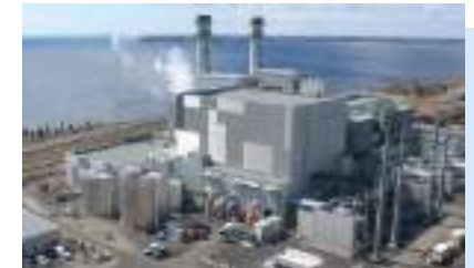
4. Napanee Generating Station Capacity 900 MW
