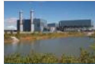
2. Halton Hills Generating Station Capacity 683 MW
