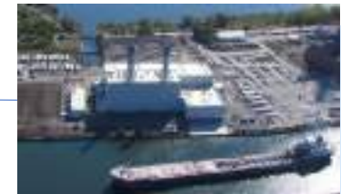
3. Portlands Energy Centre Capacity 562 MW
