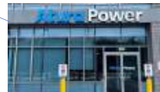
5. Oakville Head Office
