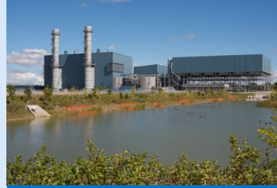
2. Halton Hills Generating Station (683 MW)
