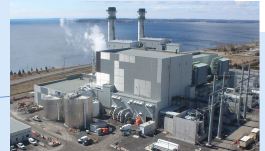
4. Napanee Generating Station (900 MW)
