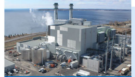
4. Napanee Generating Station Capacity 900 MW
