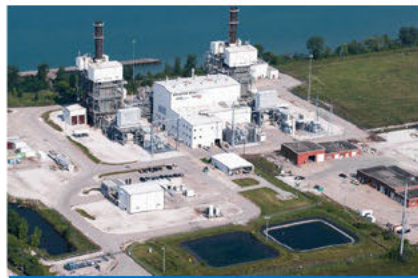
1. Brighton Beach Generating Station Capacity 570 MW
