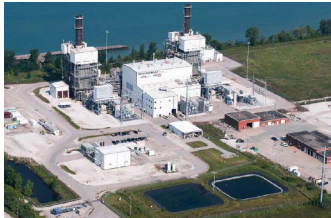
1. Brighton Beach Generating Station Capacity 570 MW
