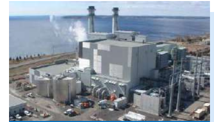
4. Napanee Generating Station Capacity 900 MW
