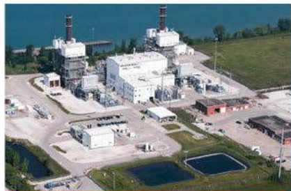
1. Brighton Beach Generating Station Capacity 570 MW
