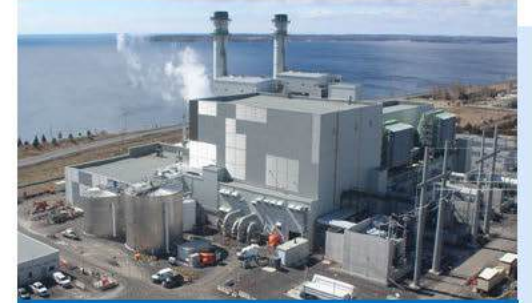
4. Napanee Generating Station Capacity 900 MW
