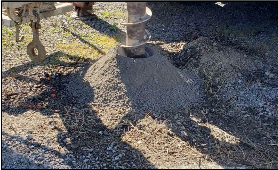
Image 66: View to northwest of gravel and other fill materials brought to surface during the drilling of borehole B-5 in Zone 5.
