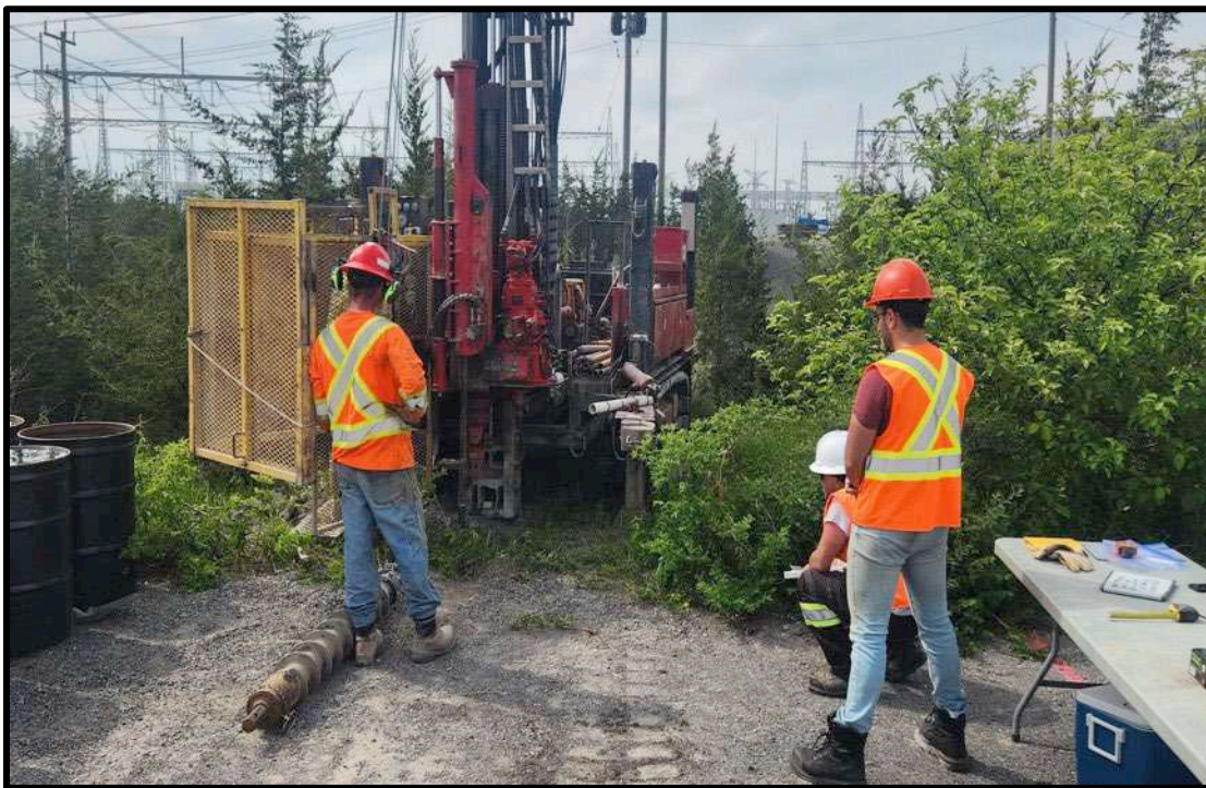
Image 50: View to west of drill rig set up to excavate borehole WH-2 in Zone 1.
