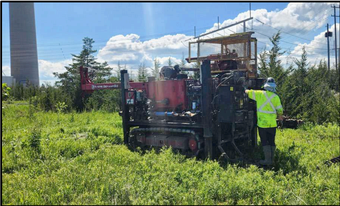
Image 52: View to west of drill rig set up to excavate borehole WH-3 in Zone 1.
