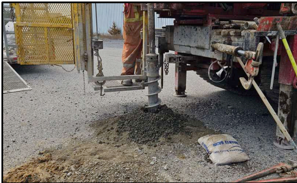
Image 67: View to northwest of the drilling of borehole B-7 in Zone 5. Note presence of sand, gravel, and rock fragments from the upper 120 cm.
