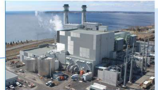
4. Napanee Generating Station Capacity 900 MW
