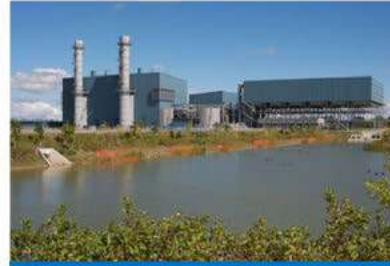
2. Halton Hills Generating Station Capacity 683 MW
