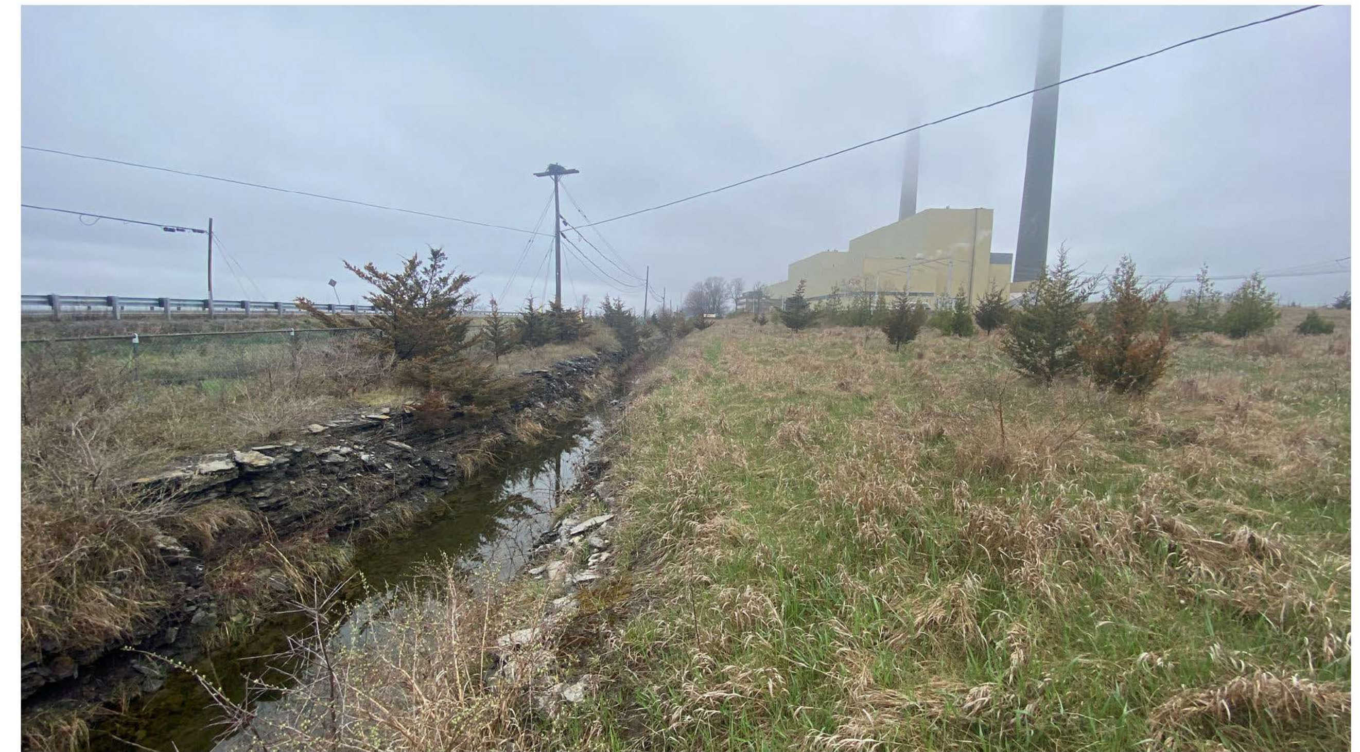
Photo of roadside drainage ditch
