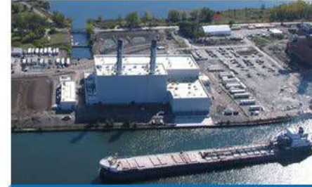
3. Portlands Energy Centre Capacity 550 MW
